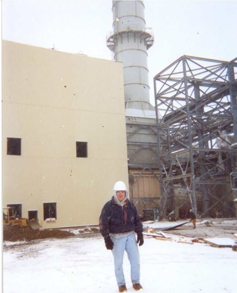
Same Combine Cycle system at different stage of installation
